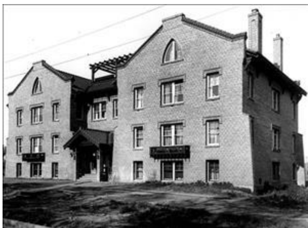
Dormitory, Washington State Normal School, Ellensburg, 1912
